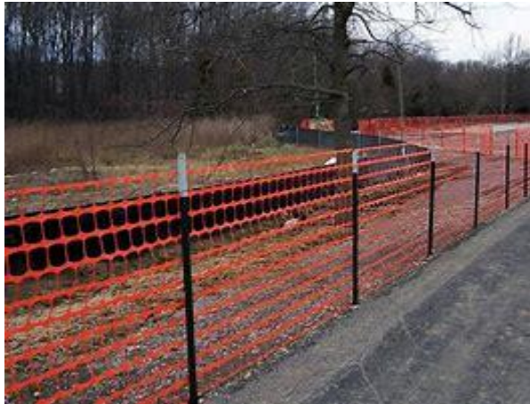
Fig. 6: Euromesh type fencing
